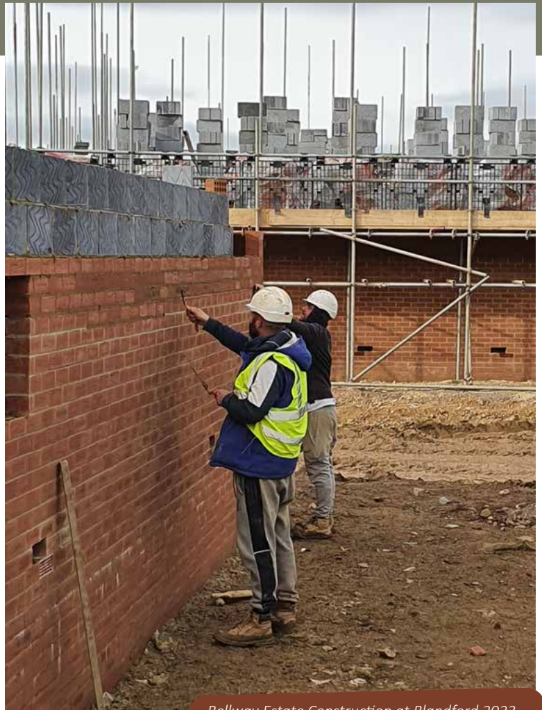
Bellway Estate Construction at Blandford 2023
