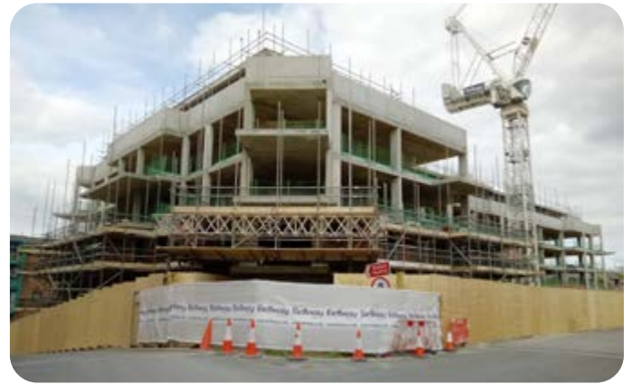
Bellway, Brewery Square development of apartments in central Dorchester
